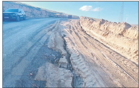
图 6 调查县区内因车辙形成的道路侵蚀 Fig.6 Road erosion caused by ruts in surveyed counties and districts
