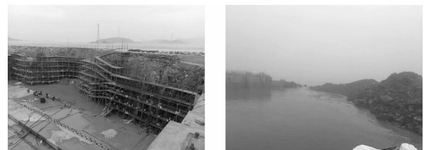
图8 爆破前后效果对照 Fig. 8 Effect comparison before and after blasting
