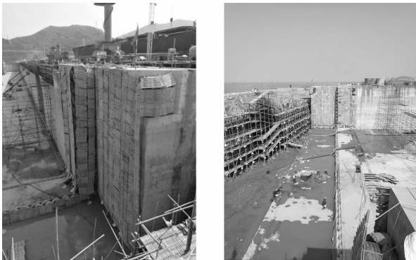
(a) 坞墩花岗岩贴面安全防护 (a) Dock pier granite veneer safety protection
