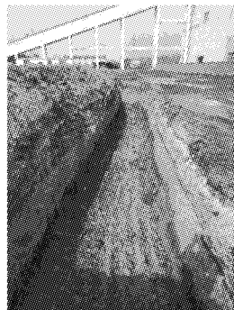
(a) 开挖减振沟 (a) Ditch of reducing vibration
