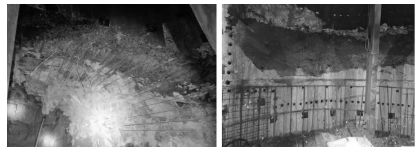
(a) 上分层施工情况 (a) Construction situation of upper layer (b) 中分层(下分层)施工情况 (b) Construction situation of middle layer (lower layer)
