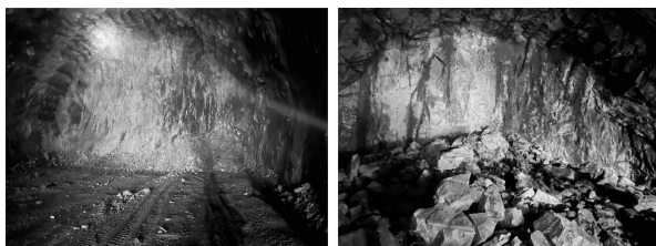
(a) 爆破后断面 (a) Blasted section
