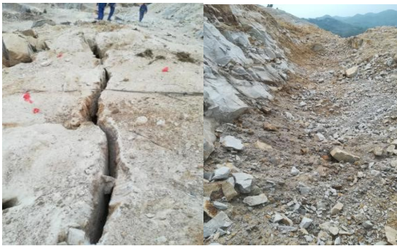
图11 爆后形成预裂缝 图12 爆后根底 Fig. 11 Pre-crack after explosion Fig. 12 Post-explosive root
