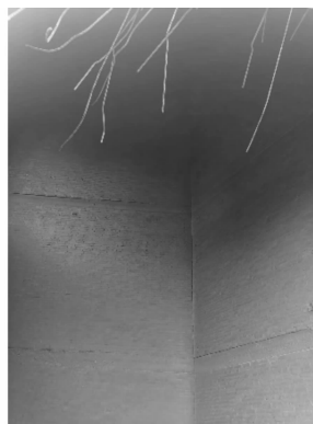
(b) Herringbone-shaped lining inside the chimney
