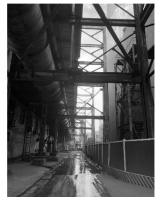
(c) Gas pipe behind the chimney
