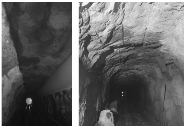
(a) 施工期 (a) Construction period (b) 竣工期 (b) Completion period
