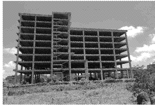
图2 楼房正面(东侧) Fig.2 Building facade(east)
