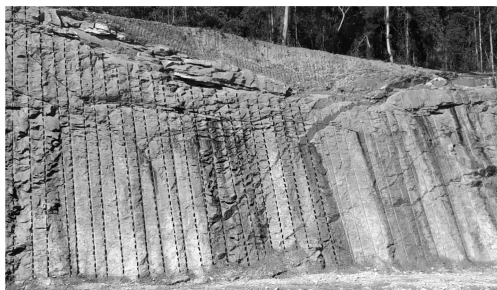
图 4 引渠段边坡深孔预裂爆破效果图 Fig. 4 Excavation effect of deep-hole presplit blasting on approach channel slope
