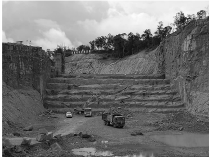
图 14 溢洪道闸室段跌坎整体开挖效果图 Fig. 14 Overall excavation effect drawing of spillway sluice chamber section drop sill
