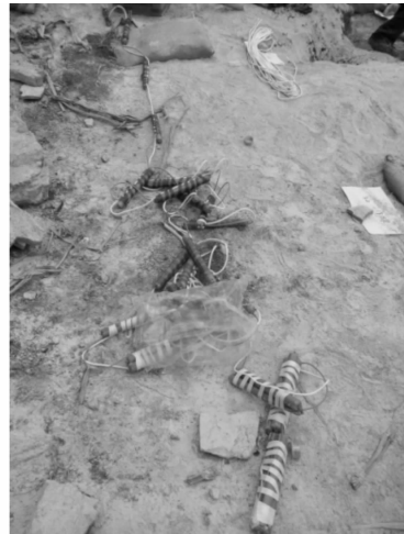
图7 光爆孔药卷 Fig. 7 Cartridge of the smooth blasting hole
