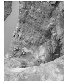
(c) 相对破碎岩体的清渣后效果 (c) Effect of relatively cracked rock mass after slag removal
