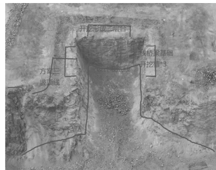
图 11 接手现状航拍图 Fig. 11 Take over the current aerial photos
