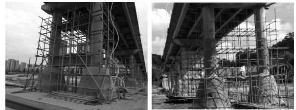
图4 排架和材料运输平台搭设示意图 Fig. 4 Schematic diagram of shelving and material transportation platform
