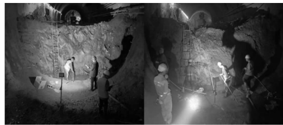
(b) 下断面爆破施工 (b) Blasting construction of the lower bench
