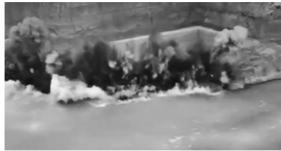
(b) 爆破瞬间 (b) During blast
