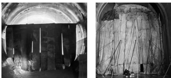
(a) 橡胶帘 (b) 机架幕墙 (a) Rubber curtain (b) Rack curtain wall
