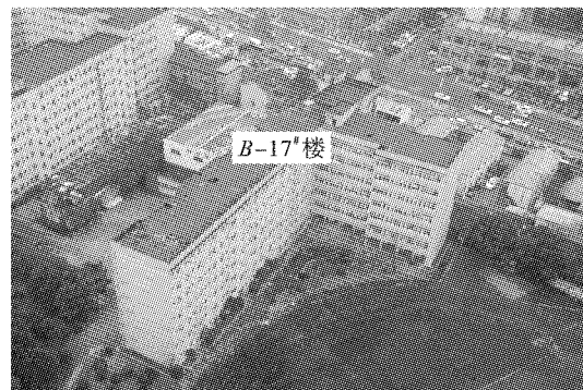
图1 待拆除B17楼
