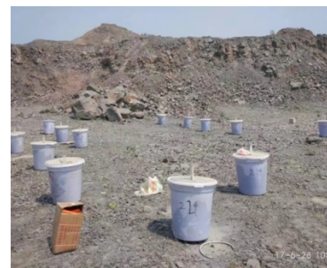
(f) 准备爆破布置 (f) Site blasting operation
