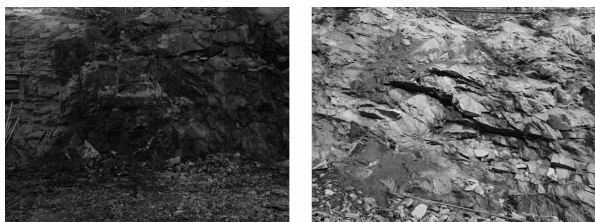
图2 硬梁包水电站开挖现场揭示地质 Fig. 2 Geology revealed at the excavation site of the Yingliangbao Hydropower Station
