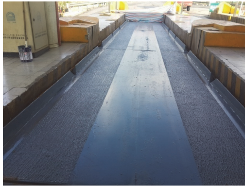
图5 高速公路用防滑涂层 Figure 5 Non-skid coating for highways
