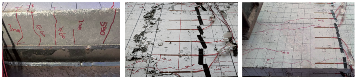
(a) 混凝土底板裂缝 (a) Cracks in concrete footings (b) 混凝土顶板贯穿裂缝 (b) Concrete roof through cracks (c) 混凝土弯剪段裂缝 (c) Cracks of concrete in bending shear section
