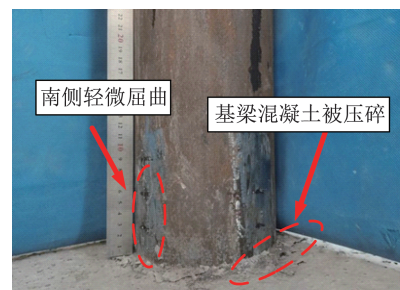
图6 试件H360-45-14-6的破坏形态 Fig. 6 Failure mode of specimen H360-45-14-6
