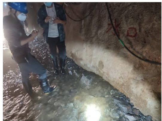
图5 小扑隧洞1#支洞YX3+657.5—668.9揭露暗河 Fig. 5 Subsurface stream exposed with the branch of tunnel 1# of the Xiaopu Tunnel at YX3+657.5—668.9
