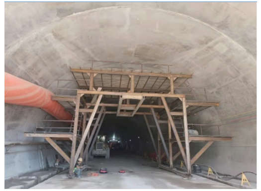
图 3 隧道现场情况 Fig.3 On-site conditions of the tunnel
