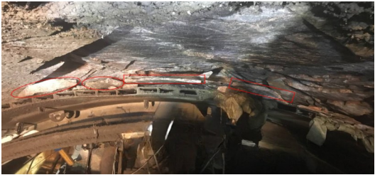
图 7 强岩爆在盾体上方产生的岩块 Fig. 7 Rock elements produced by strong rock burst in the real site
