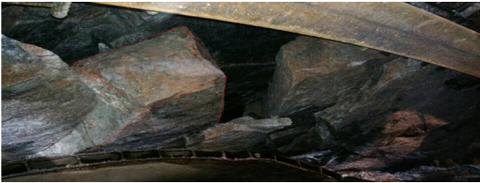
图 8 极强岩爆在盾体上方产生的岩块 Fig. 8 Rock elements produced by extremely strong rock burst in the real site
