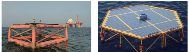
图2 中国海上FPV案例 Fig. 2 Cases of offshore floating photovoltaic structures in China
